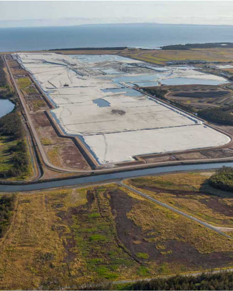
For the Brisbane Airport, Australia, we reclaimed a 300-hectare platform for the construction of a new runway.
