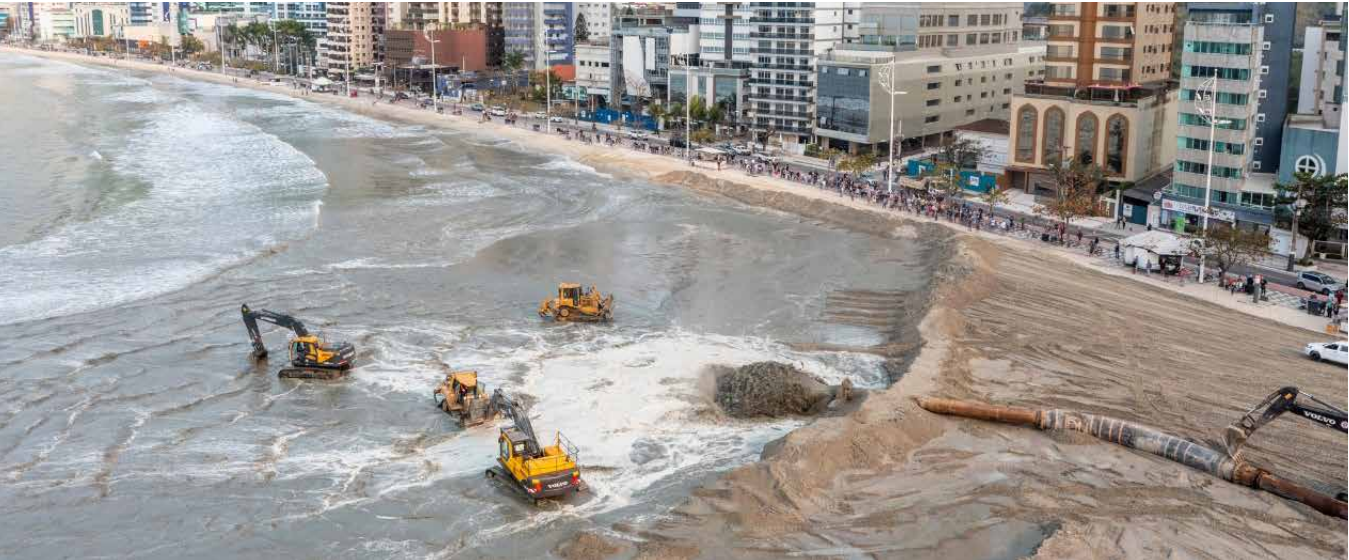
In nine weeks' time, we expanded 5.8 km beach in the Brazilian coastal city of Balneário Camboriú to counteract erosion, create more beach, and protect coastal roads from violent storms and tides.
