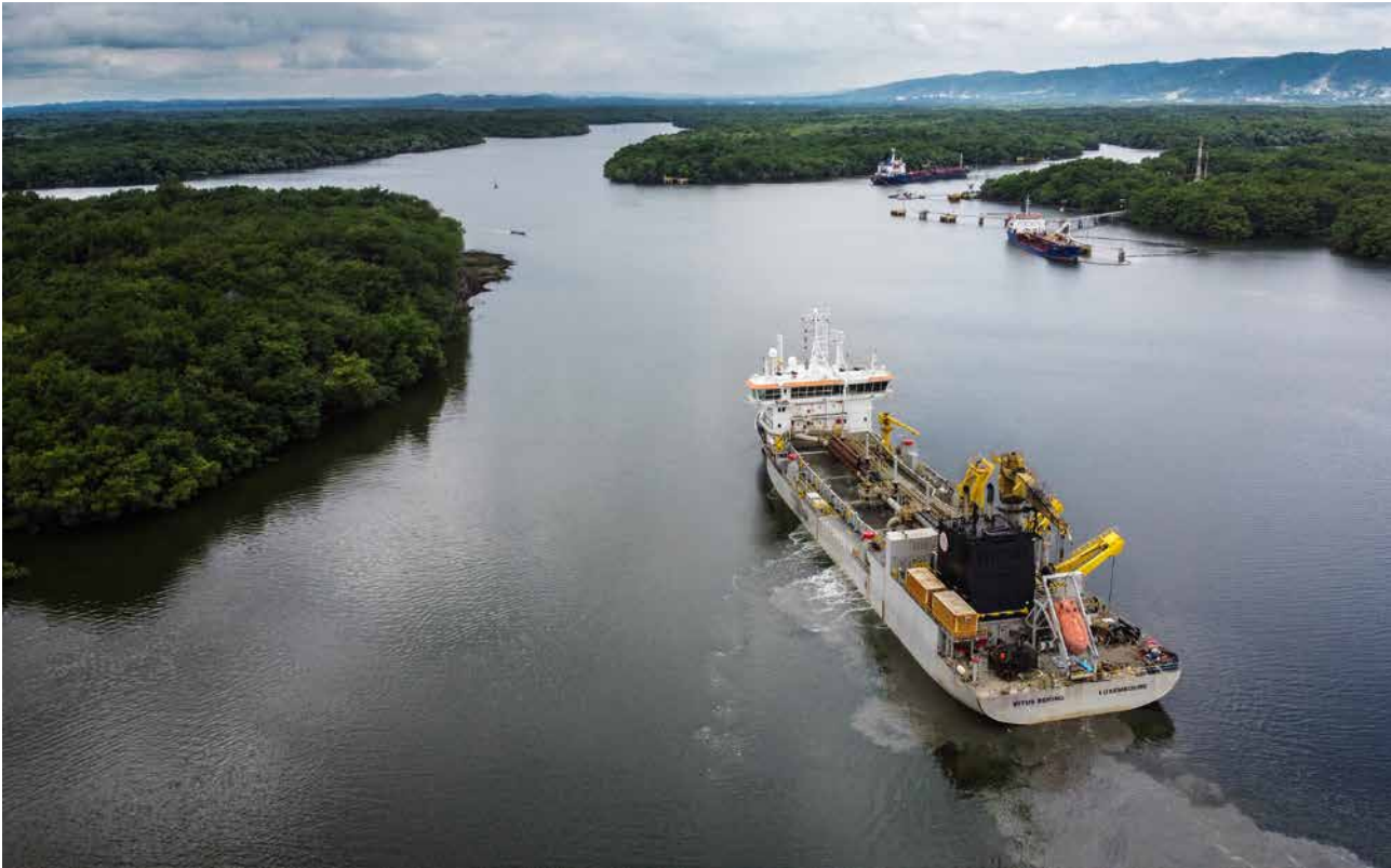
To keep the port of Guayaquil, Ecuador, accessible to Neo Panamax and other large vessels, we deepened its access channel to 12.5 metres.
